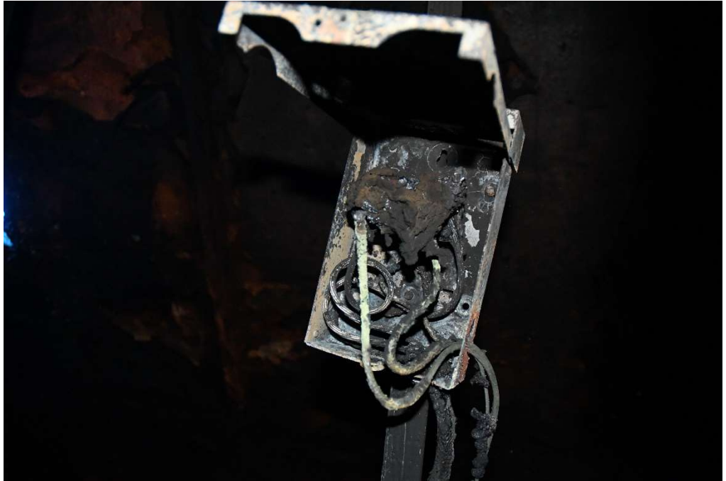
Disconnect in fire damage condo
