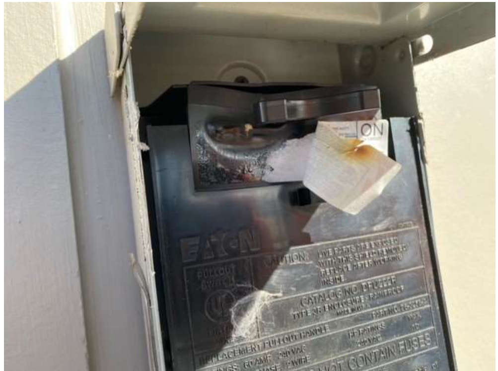
Melted pull-out handle
